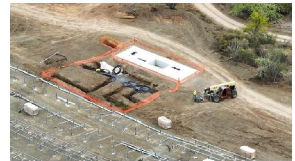
PI – INVERTER STATION FOUNDATION
