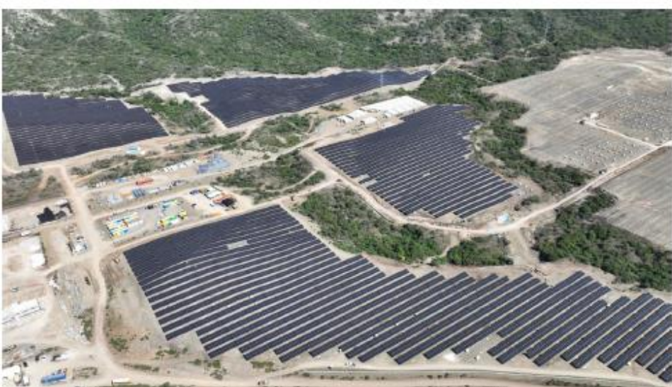
PII – PILLING / MODULE INSTALLATION WORKS
